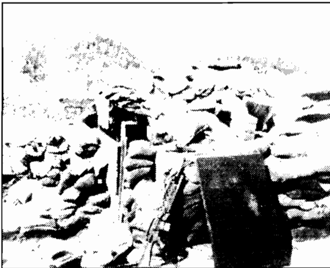
An M-203 rests against a caved-in bunker, one of many structures destroyed in the NVA's early morning attack on March 28, 1971. The soldier who had carried the rifle-grenade launcher combination perished inside.
